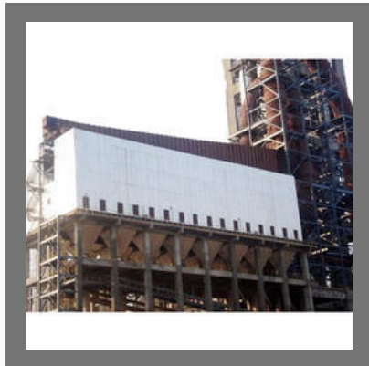
Hot Gas Electrostatic Precipitator
