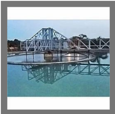
WTP Designing Service
