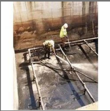
WTP Erection & Commissioning Services
