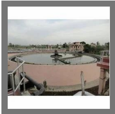
ETP Operation And Maintenance
