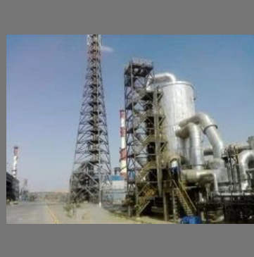
DM Plant Erection Services
