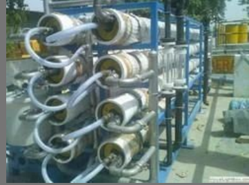
ETP Erection And Commissioning Services
