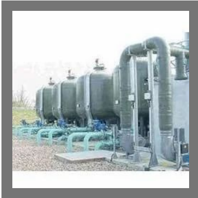
WTP Engineering service
