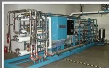
Softener Commissioning Service
