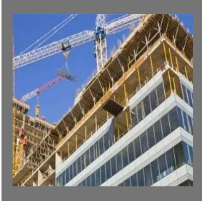
Commercial Civil Work Service
