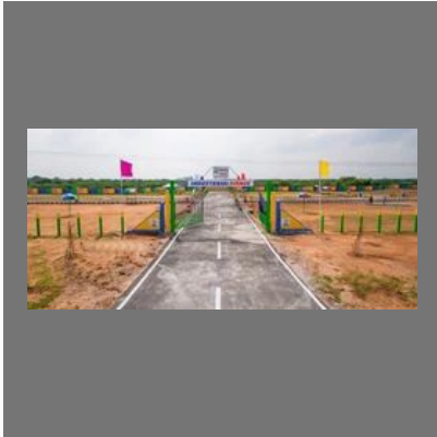
Industrial Avenue Service
