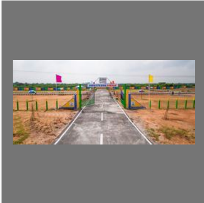
Industrial Avenue Service
