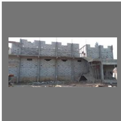
Solid Concrete Bricks Building
