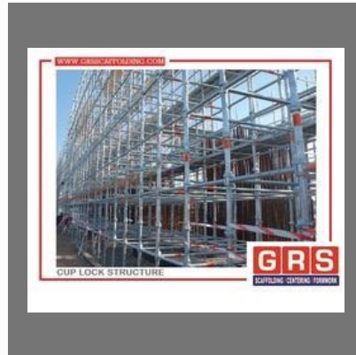
Structure Scaffolding Cup Lock
