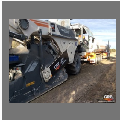
Advanced Soil Stabilisation Service
