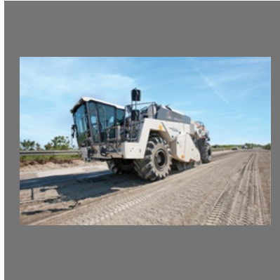
Cement Treated Base Service
