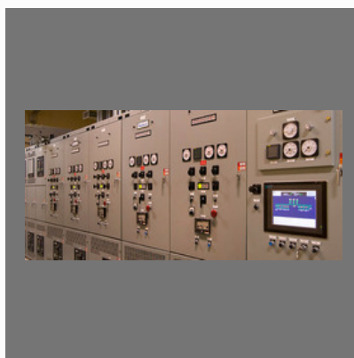
Switchgear Panel
