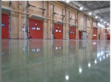
Industrial Super Flat Floors Construction Service
