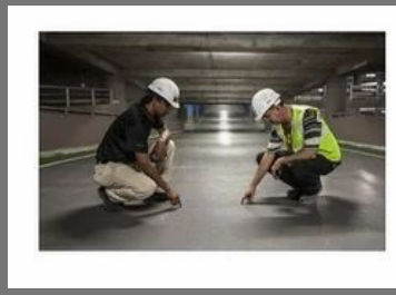
Steel Fibre Reinforced Concrete Flooring
