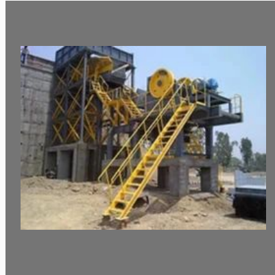
Stationary Crushing Plant
