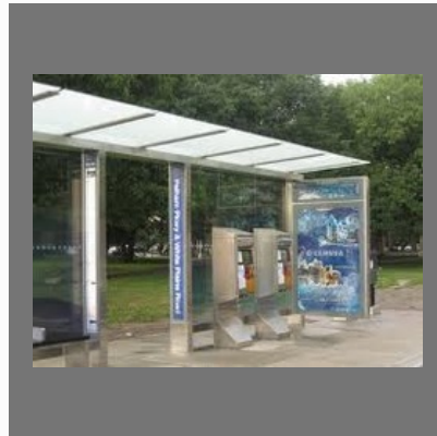
Bus Shelters Services
