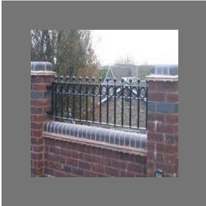
Boundary Wall Railing
