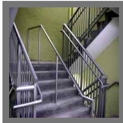
Stair Case Railing
