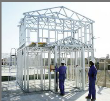
Light Steel Structure
