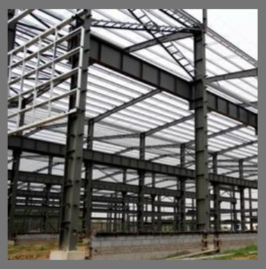
Heavy Steel Structure
