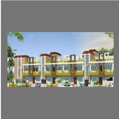
Residential Apartments Construction
