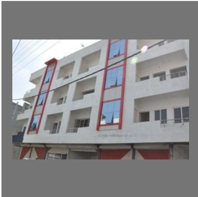
Apartment Construction Service
