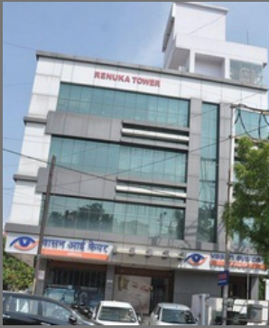
Tower Construction Service
