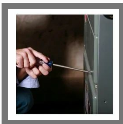
Furnace Maintenance Service
