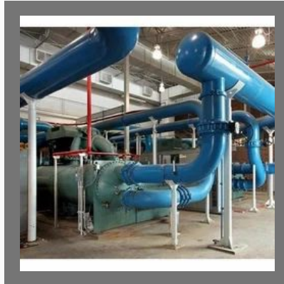
Water Utility Piping Turnkey Projects
