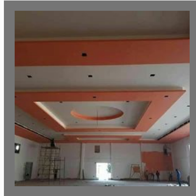
Gypsum Ceiling Work
