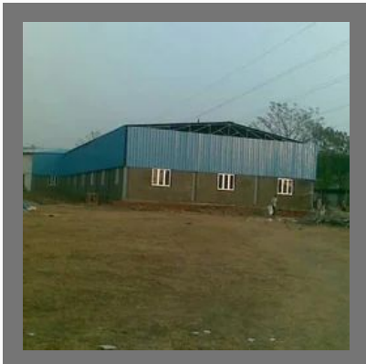
Prefabricated Factory Shed
