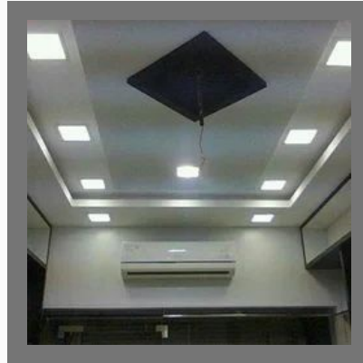
Gypsum False Ceiling
