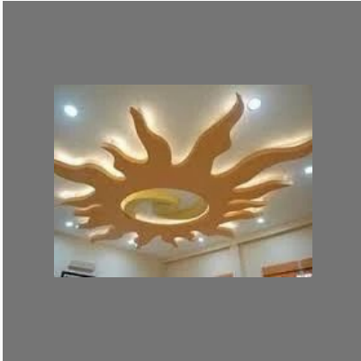
Gypsum False Ceiling
