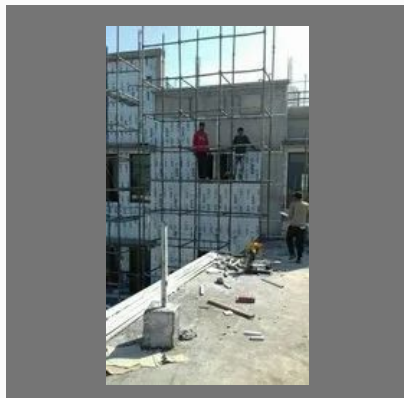
Aluminum Composite Panel Fabrication Work
