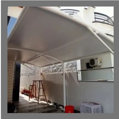
Car Parking Shed Work
