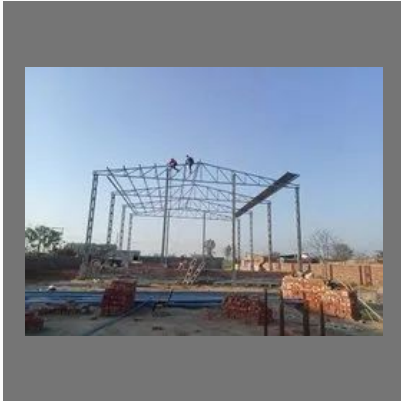
Iron Industrial Fabrication Shed
