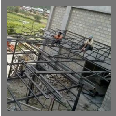
Industrial Steel Shed
