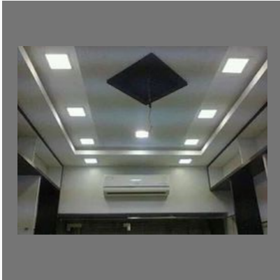
Gypsum False Ceiling
