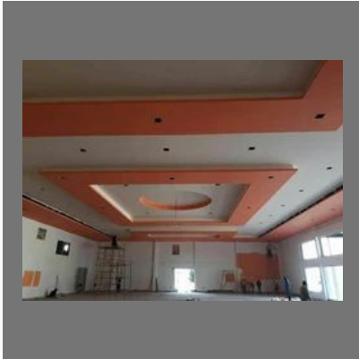
Gypsum False Ceiling
