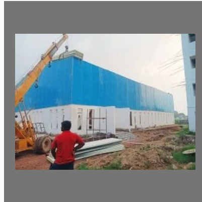
Warehouse Metal Sheds
