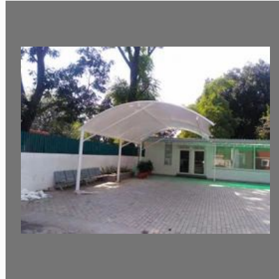
Water Proof Shed
