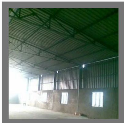
Modular Steel Warehouse Shed
