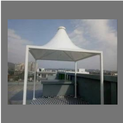
Auditorium Tensile Structure
