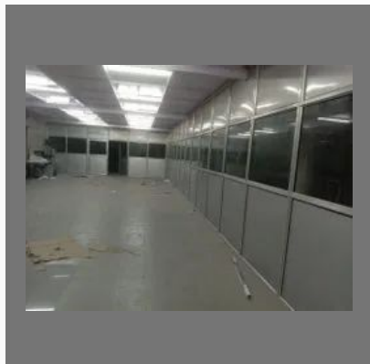
Aluminium Fabrication Glass Work
