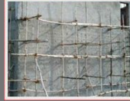
Injection Grouting
