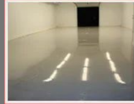
Epoxy Flooring And Coating 01
