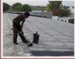
Bituminuous Coal Tar Waterproofing
