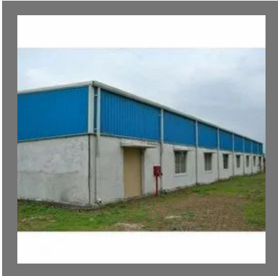
Warehouse Industrial Shed
