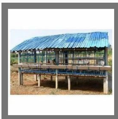
Mild Steel Poultry Farm Shed
