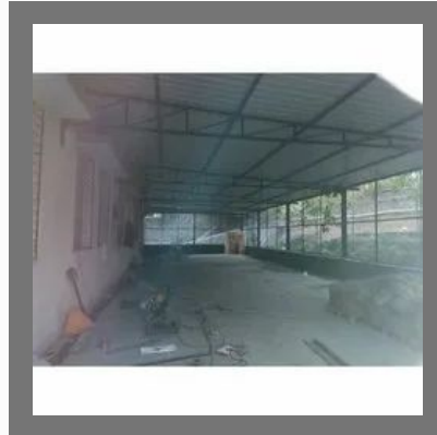
Industrial Godown Structural Fabrication
