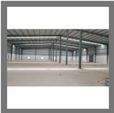
Mild Steel Industrial Shed
