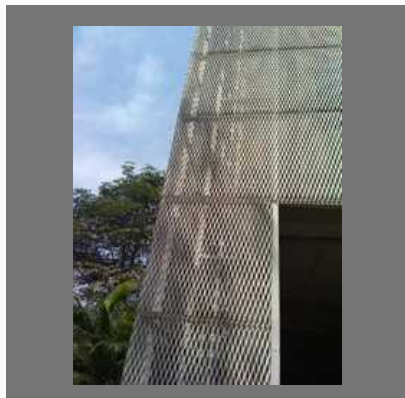
Aluminium Jali Building Shed
