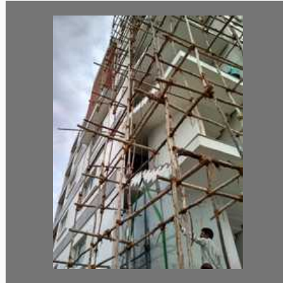
Aluminium Building Works
