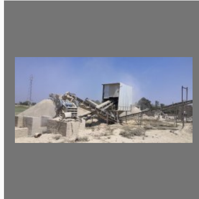
Jaw stone crusher plant
