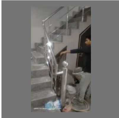
Stainless Steel Staircase Railing
