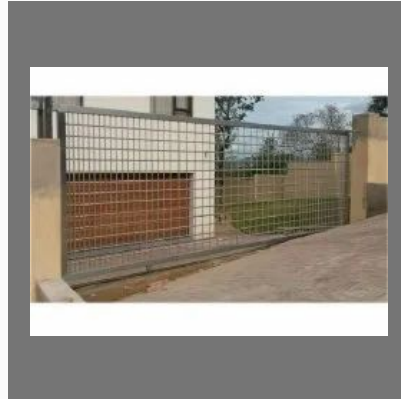
Commercial SS Main Gate
