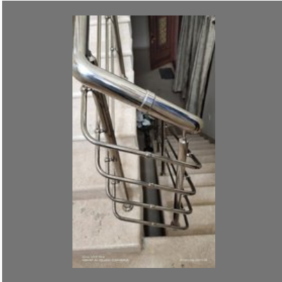
Ss Staircase Railing
