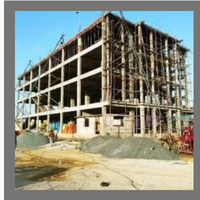
Building Construction Services
