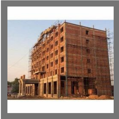
Hotel Building Construction Services
