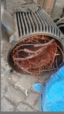
Paper Mill Motor Repairs
