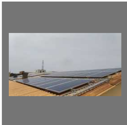
Solar Panel Installation
