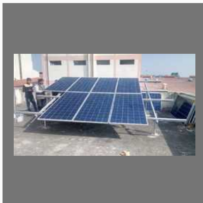
Solar Panel Installation
