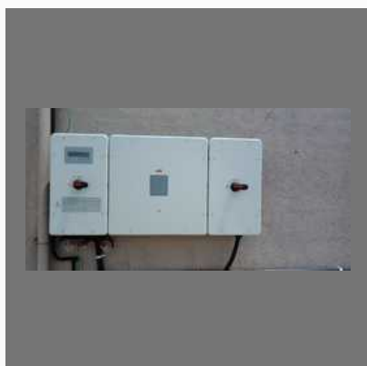
Solar Panel Installation
