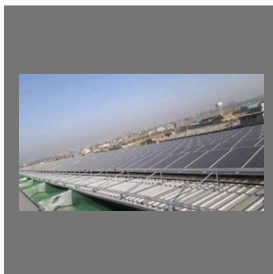
Solar Panel Installation
