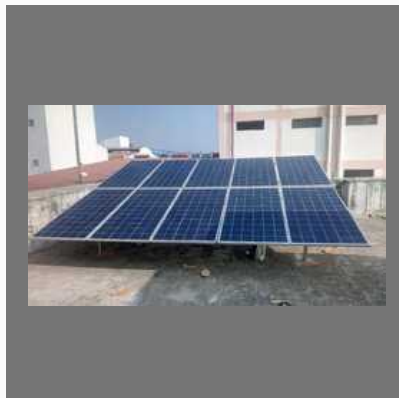
Solar Panel Installatio
