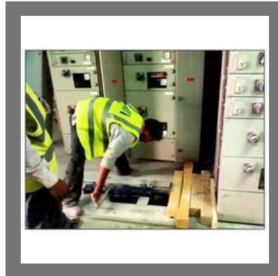
Panel Installation Service
