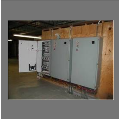
Electrical Panel Installation
