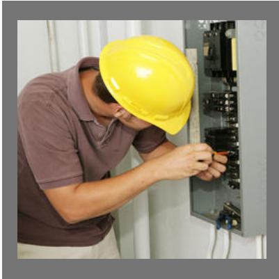
Electrical Contracting Services
