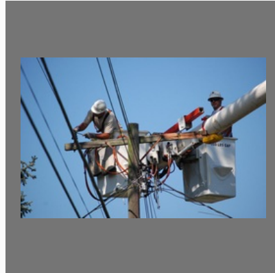
Electrical Substation Installation Services
