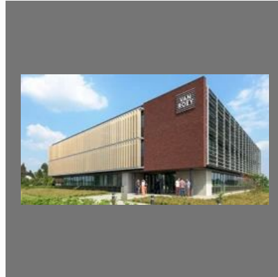
Office Construction Service
