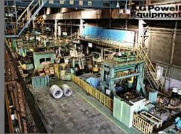
Coil Build-up Lines
