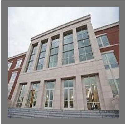
School Building Construction Services
