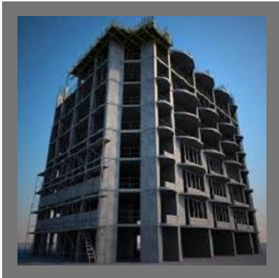
School Building Construction Services
