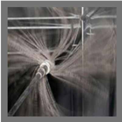
HVAC Duct Cleaning Service
