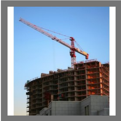
Site Inspection Service
