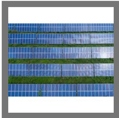
Solar PV module Inspection Service by Thermal camera Drones.
