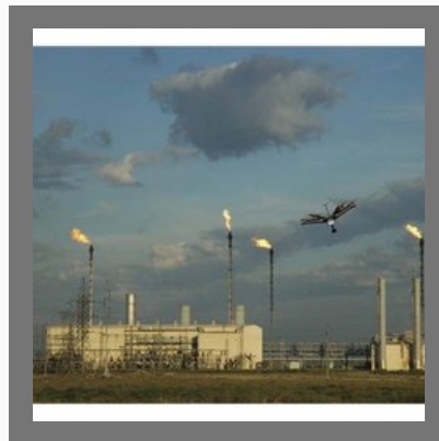
Stack and Flare Inspection
