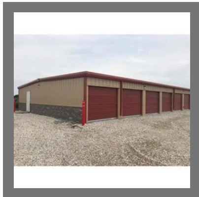
Pre Engineered Warehouse Building
