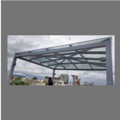
Ms Canopy Structure
