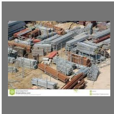
Steel Stack Yard
