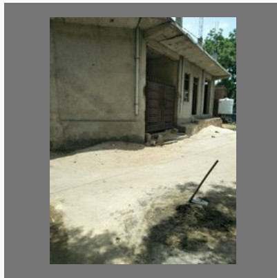
School Building Construction Services
