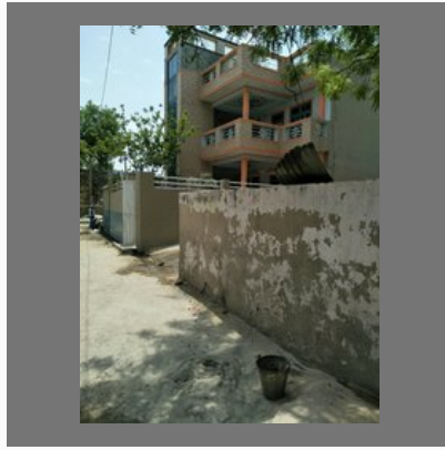
Commercial Building Construction Services
