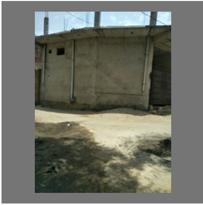
Industrial Building Construction Service
