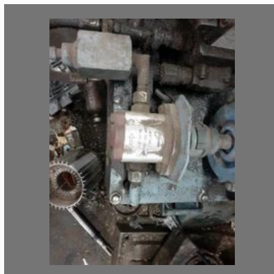
Hydro Pneumatic Pump Repairing
