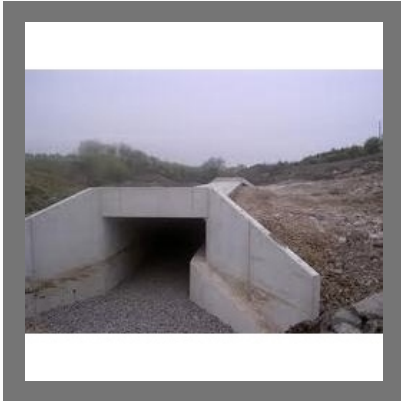
Concrete Bridge Culverts
