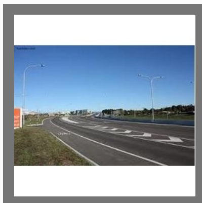
Bridge Approach Roads
