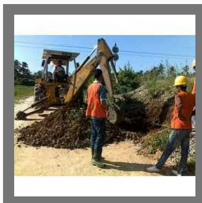
Civil Maintenance of Building
