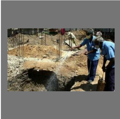
Pre-construction Termite Service
