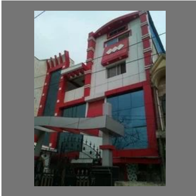
ACP Sheet Fabricated Structure
