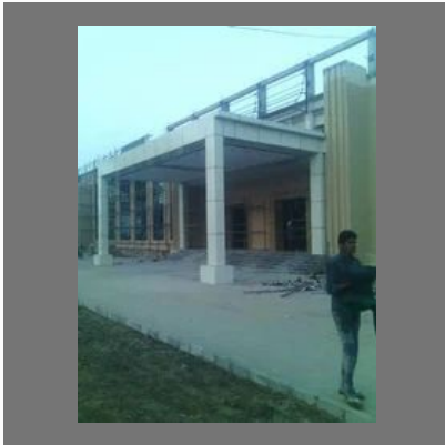
ACP Fabricated Structure
