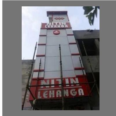
ACP Sheet Structure
