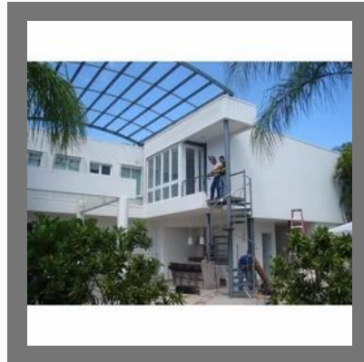
Residential Steel Fabrication Service
