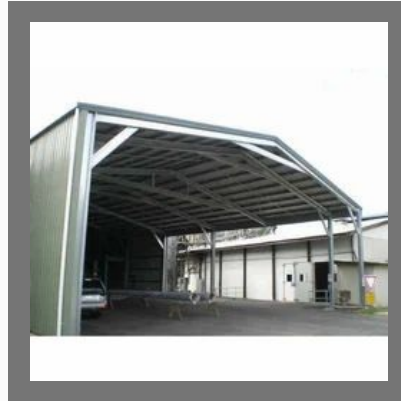
Polycarbonate Industrial Shed
