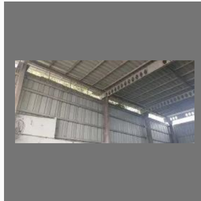
Work Shop Shed Work
