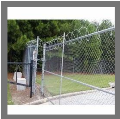
Mild Steel Wire Net Fencing Work
