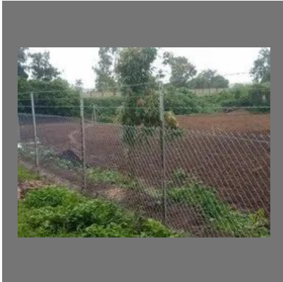
Weld Mesh Net Fencing Work
