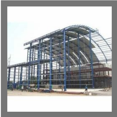
Industrial Shed Fabrication Service
