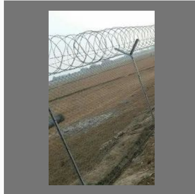
Chain Link Net Fencing Work
