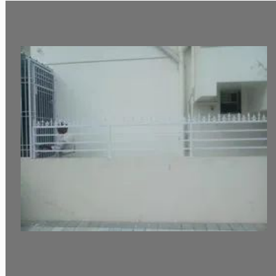
Compound Wall Railing Work
