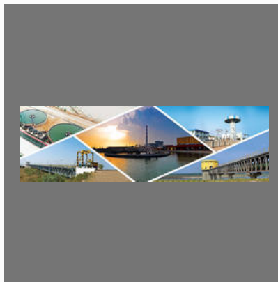
Industrial Building Consultancy Service
