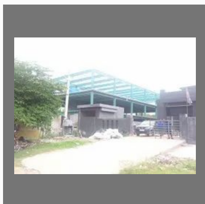
pre engineered building works
