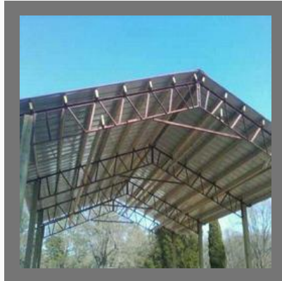
Industrial Shed Structural Fabrication Service
