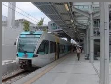
Airport And Railway Station
