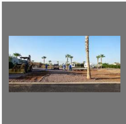
Fitness Center (Project In Progress)
