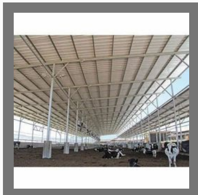
Dairy Roofing Shed
