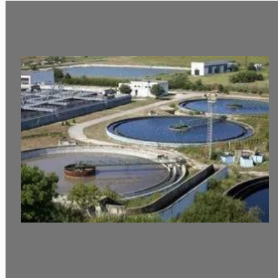
Automatic Industrial Effluent Treatment Plant
