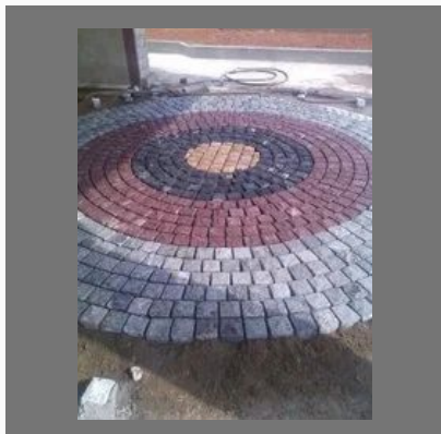
Cobble Stones Laying
