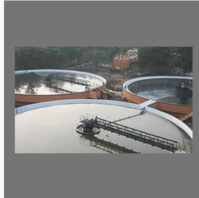
Centralized Scada System For All Sewage Treatment Plants
